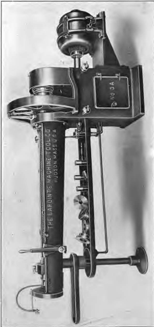
Fig. 9.—Broaching machine with motor drive.
